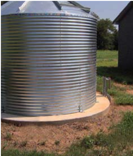
RAIN WATER HARVESTING SYSTEM
